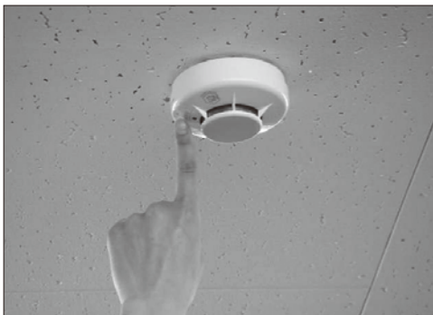
※ Photo of a smoke detector.
